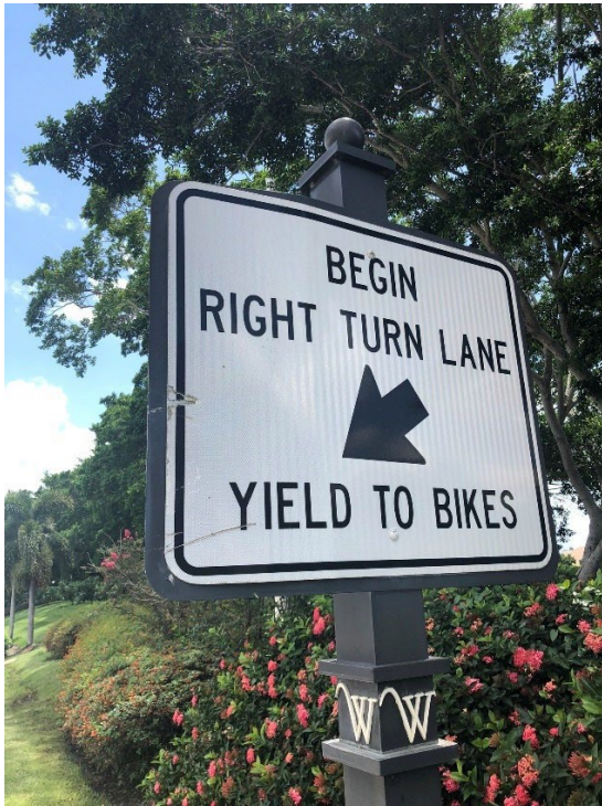
Figure 3.5-B– Typical Damage to Sign Blades and Back Plate
