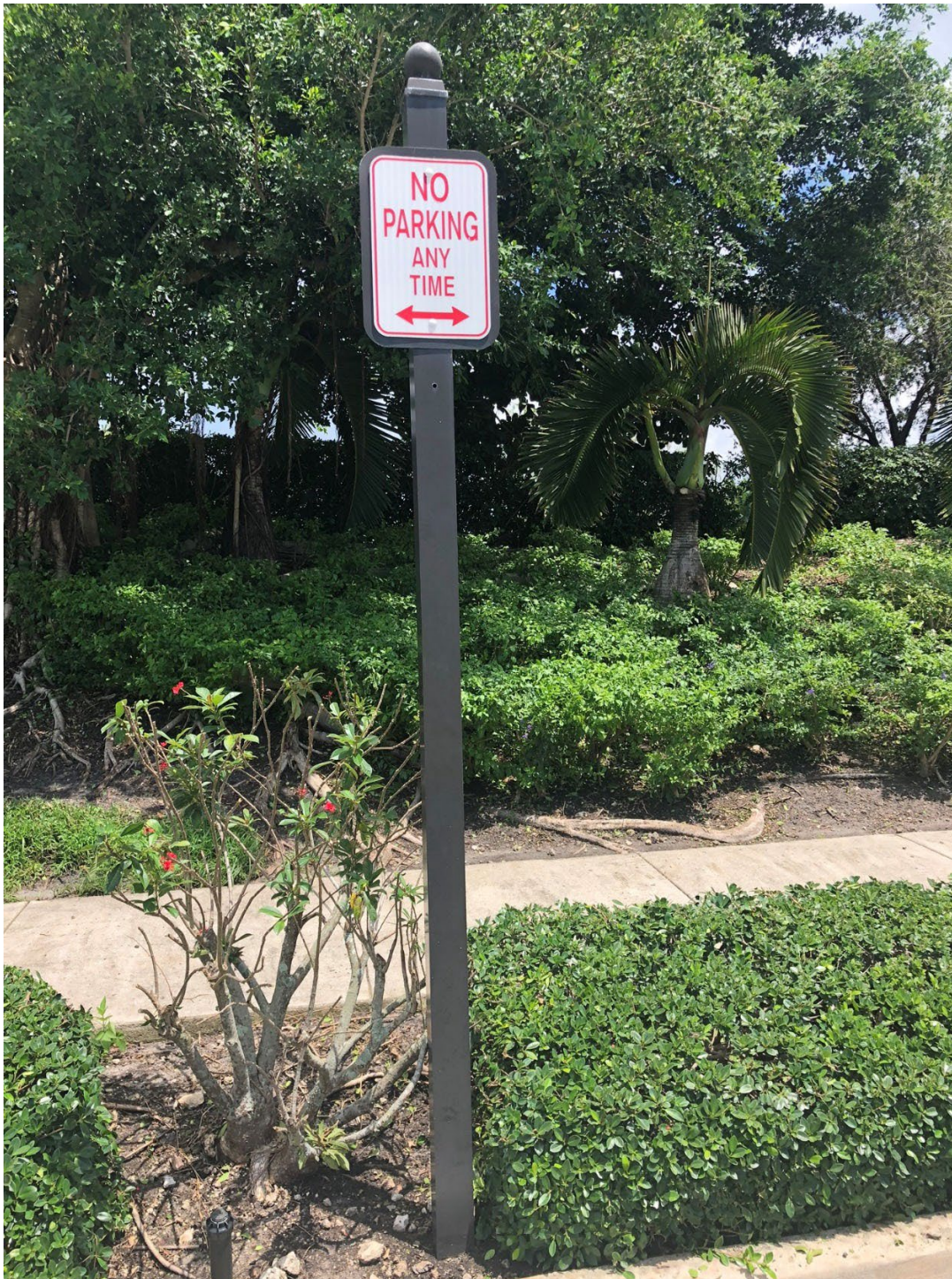
Figure 3.4-F– Type F - 4"x4" Plain 12'-0" High Post (No collars, No outer base, No "W")
