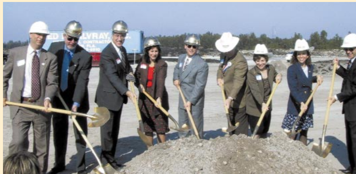
Shovels in hand, ground is broken and construction began on Weston's newest Elementary School, School "P".
